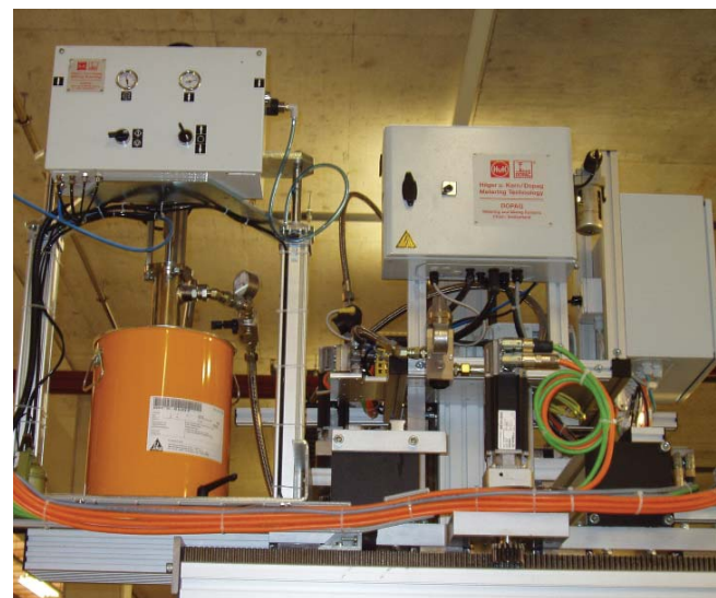
The DOPAG P30 pump and gear metering pumps are mounted overhead, directly above the robot stations
